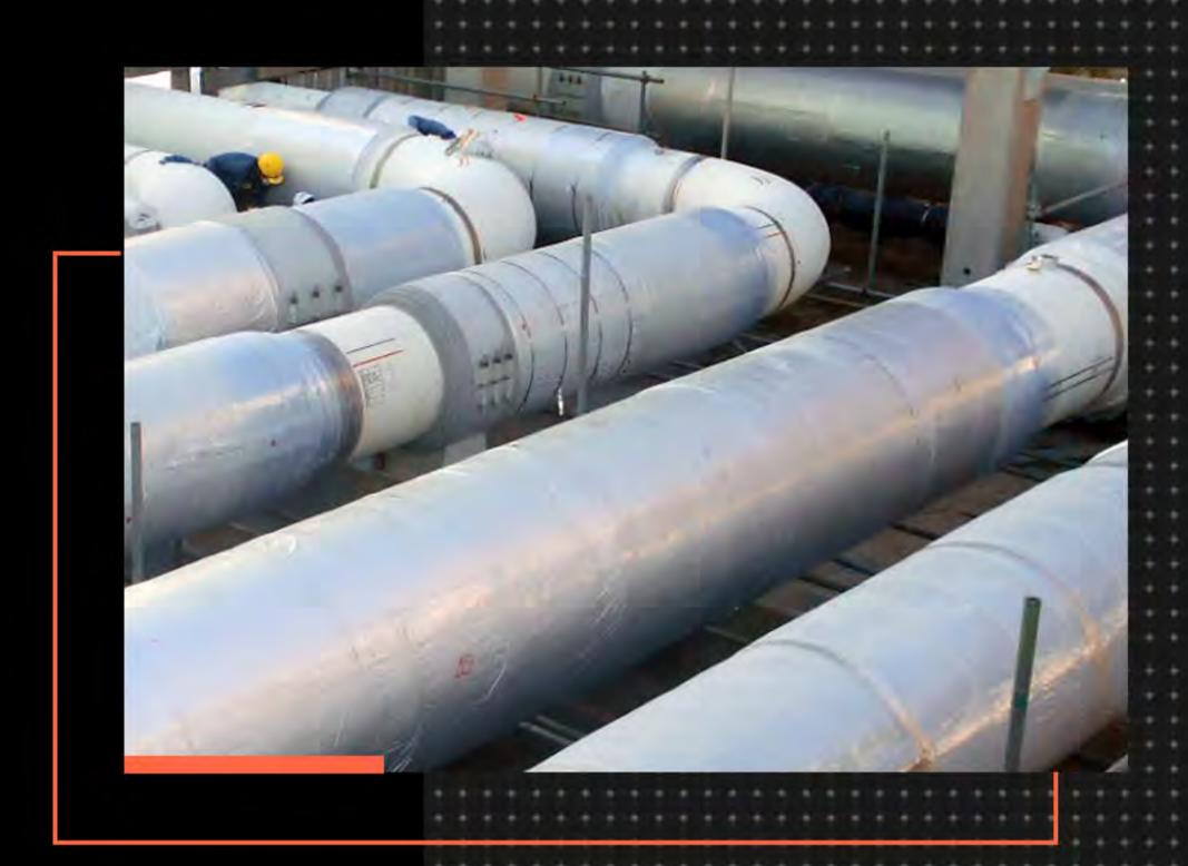
Cryowrap pipe supports, manufactured with Cryogel insulation material, provide the complete solution for supporting and restraining pipe in low temperature applications.
